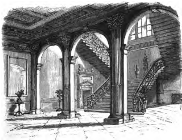
STAIRCASE OF CHESTERFIELD HOUSE.
